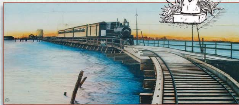
Postcard Of The Old Rail Road Bridge. This Is Reproduced As A Mural At Caroline Street.
