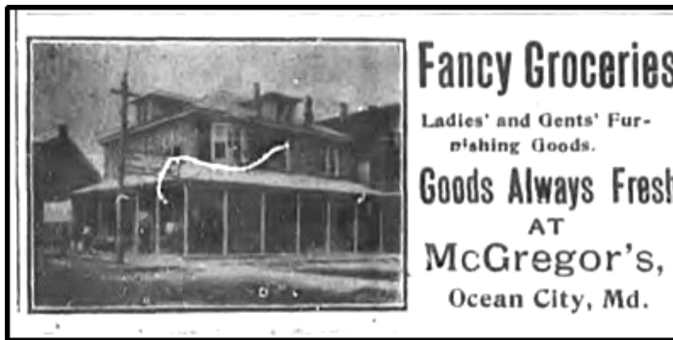
Figure 1: The McGregor Building in Ocean City. The Berlin Advance , July 28, 1911.
