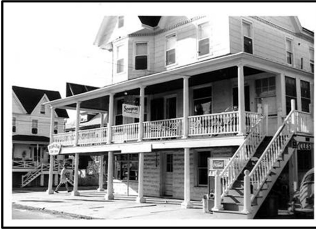
The former "Scott House" as it appeared in 1966, viewed from Caroline Street.
