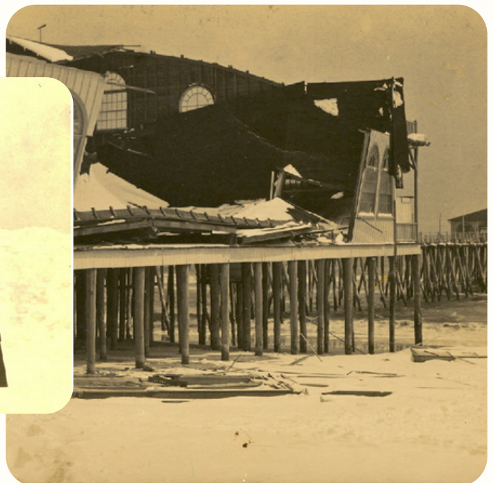
STORM of 1917: Pier building collapse from snowstorm in 1917. Collection of Violet Davis.
